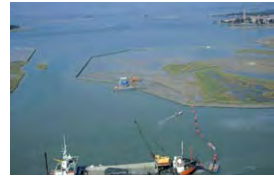
Figure 5: the realization of artificial morphological structures. STAGE 0: mixtures of sediment and water flowing into the delimitations. Even in this first phase these areas are suitable feeding and nesting sites for avifauna.
