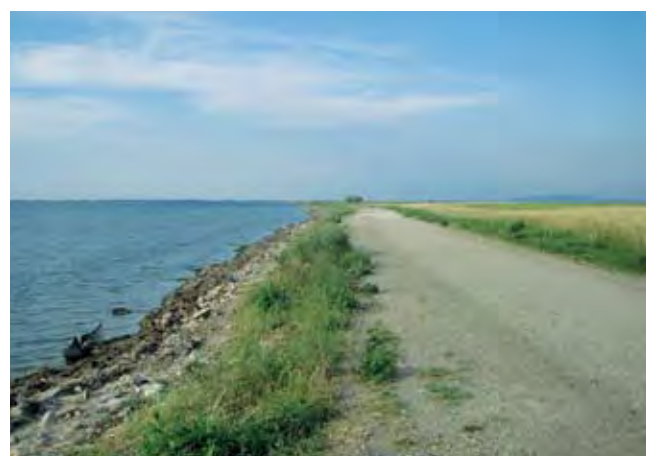
Figure 6: view of the southern bank. The dike upon which the road runs was initially part of reclamation works carried out to prevent flooding of the bordering land.
