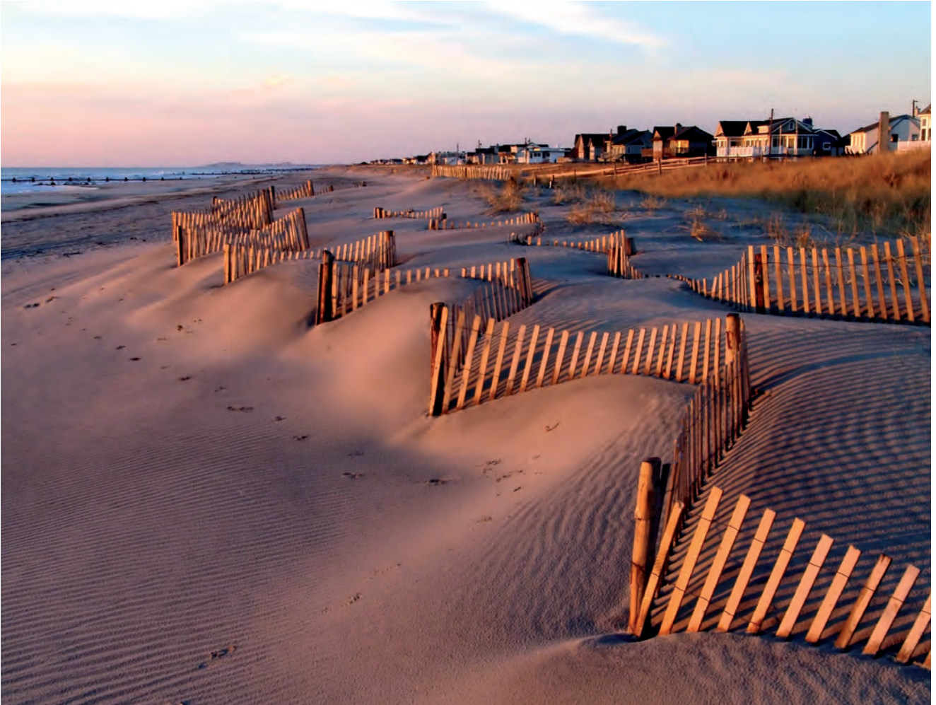
Figure 6a: double row zigzag windbreak structures, Stone Harbor, New Jersey. (picture: www.flickr.com ; Photo: Makz, 2006).
