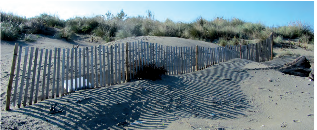
Figure 6b: brush windbreaks positioned at the foot of existing dunes to intercept the Bora wind transport blowing across the coastline (Alberoni, Venezia). (Photo: A. Bonometto, 2012).
